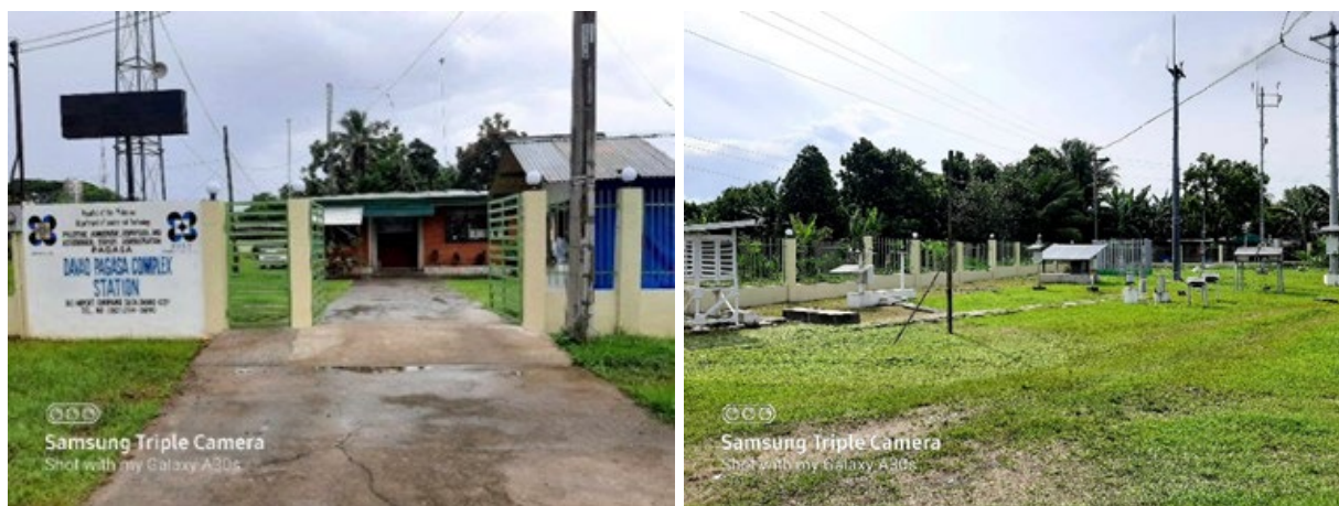
Figure 8. Davao Complex Station. (left) Facade (right) Observation Garden
