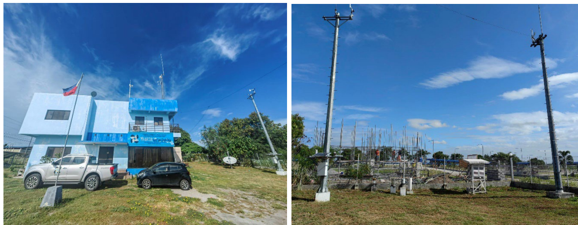
Figure 10. General Santos Station. (left) Facade (right) Observation Garden
