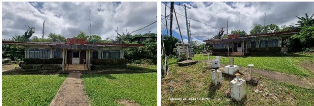
Figure 14. Surigao Synoptic Station. (left) Facade (right) Observation Garden
