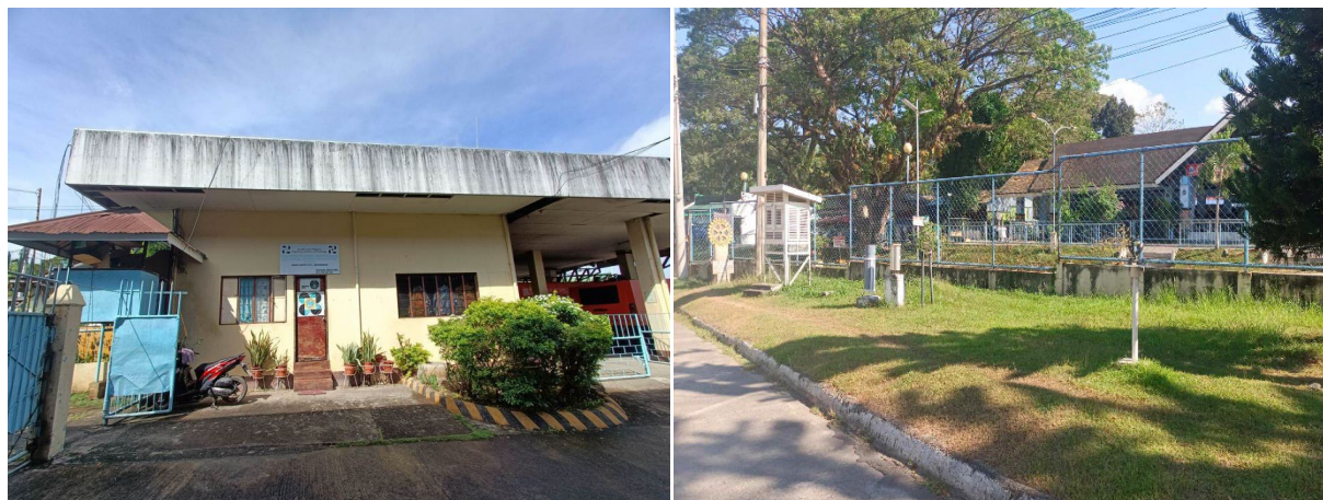
Figure 7. Facade (left) and Observation Garden (right) of Cotabato Station
