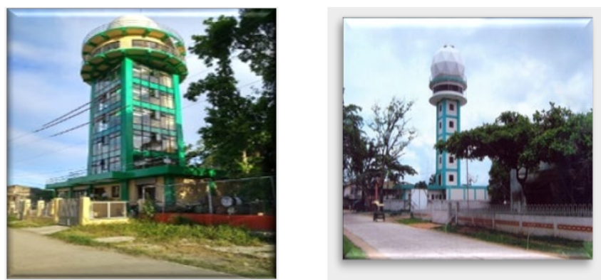
Figure 5. Zamboanga (left) and Hinatuan (right) Radar Stations
